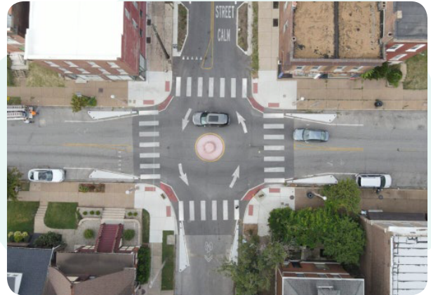
Louisiana calm streets project
